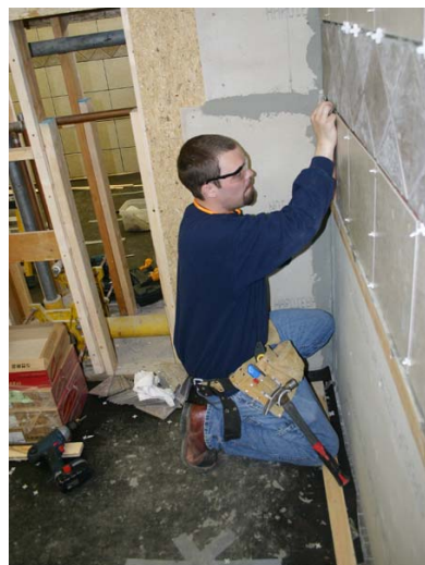
HBI student Frank Vojkuska tiles the walls of the Academy restrooms now under renovation by students.
