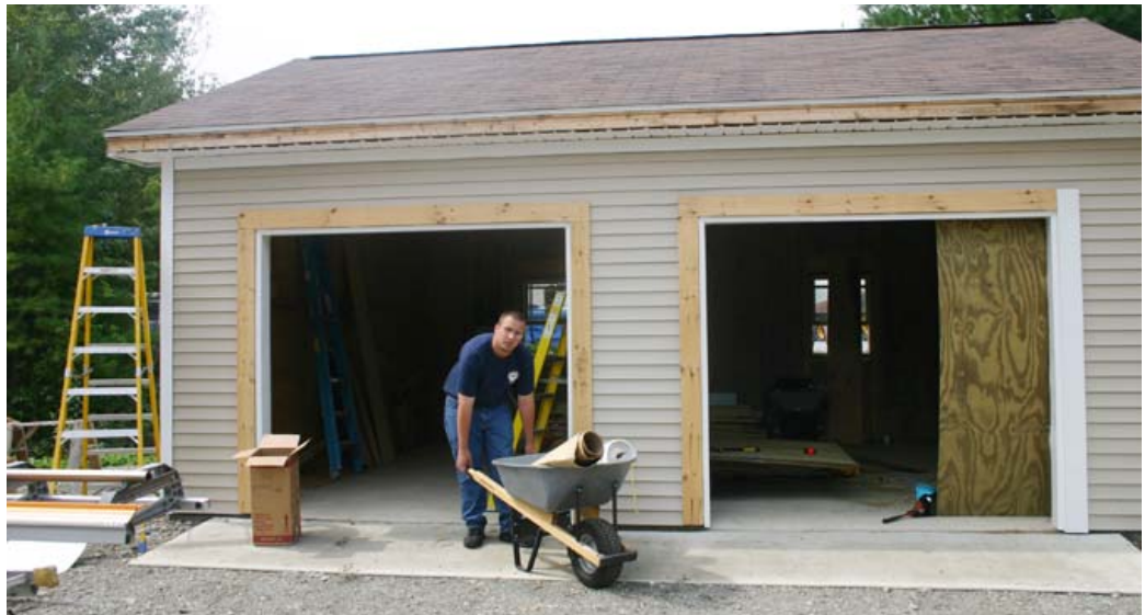
PJCA Facilities Maintenance students like Ambassador Zackery Terrio (working above) use their career skills from the Home Builders Institute classroom to construct a two-bay garage at the Academy to house the new electric maintenance vehicles.
